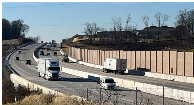
Traffic moves along the improved section of Interstate 78 in eastern Berks County. EVAN JONES/THE MORNING CALL
